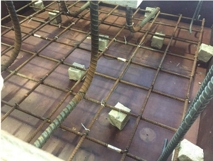
Typical Spread Footing
