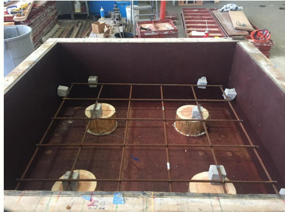
Typical Timber Pile Footing
